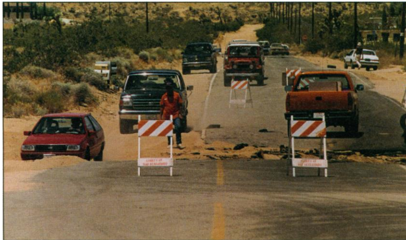
Shifting science. An earthquake that struck in 1992 caused this rupture, which shifted Reche Road in Landers, California. After the rupture, the edge of the far section was aligned with the center line of the near section. Knowledge of how such earthquakes are initiated may reveal whether the existence of a preparatory stage could be used for earthquake prediction. [AP/Wide World]
