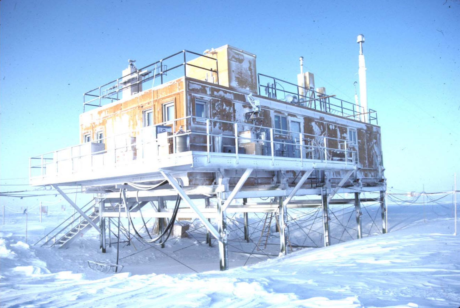
Clean Air Facility at South Pole Station, March 1992
